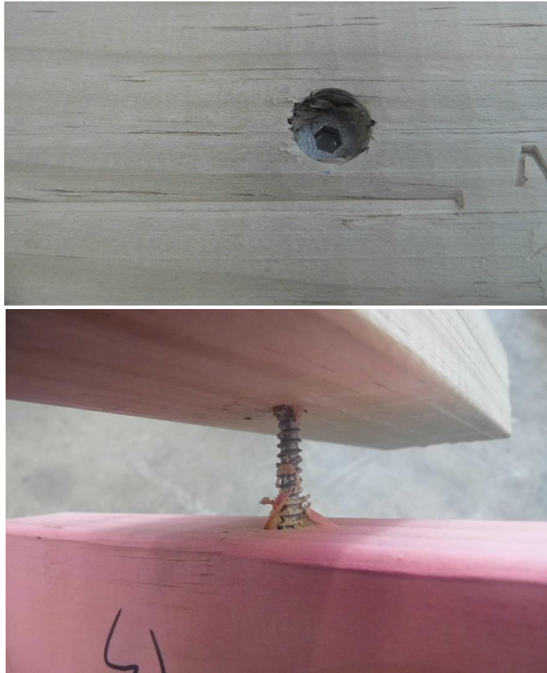
Figure 3. Examples of Screw Failures: Screw-Head Pulling Through Batten (Top) and Screw Thread Withdrawal from Purlin (Bottom)
